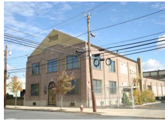
Two Story Office, 13,565 SF
