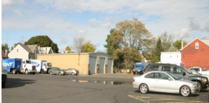
Repair Facility, Bldg. 4
