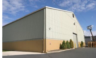
Rear Bldg. 3, 44,574 SF, Clear Span
