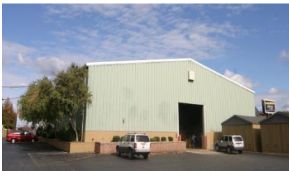
Rear Bldg. 1, 12,200 SF, Clear Span
