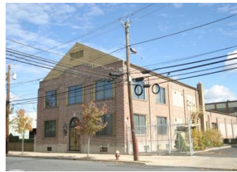
Two Story Office, 13,565 SF
