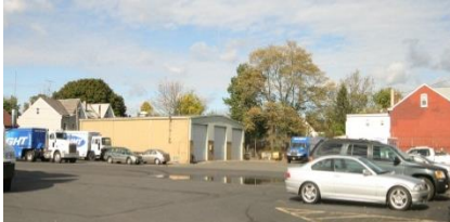
Repair Facility, Bldg. 4
