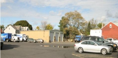
Repair Facility, Bldg. 4
